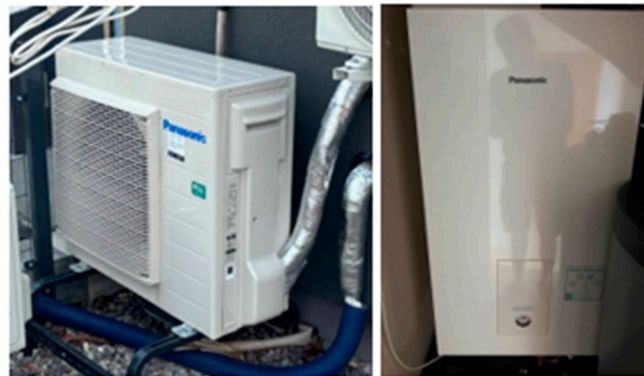
Figure 3. Air-to-water heat pump.
