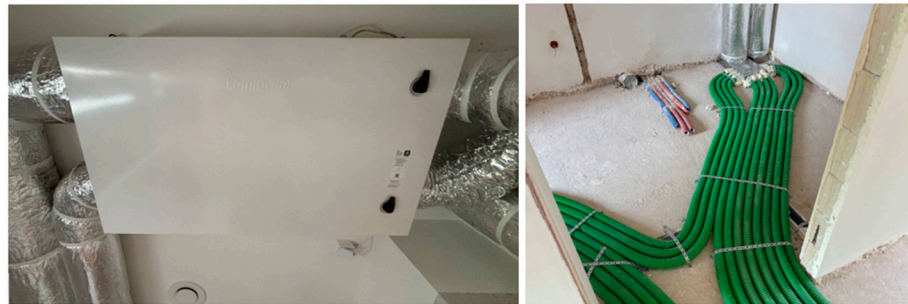
Figure 5. Komfovent heat recovery unit and HRV installations.
